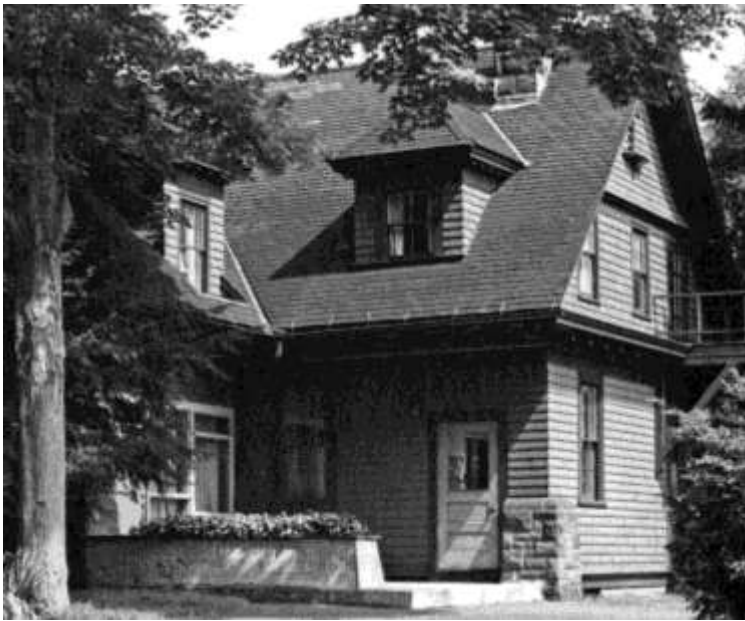
Converted carriage house at rear of the former Shaffer property — 704 Whitney Avenue, New Haven
